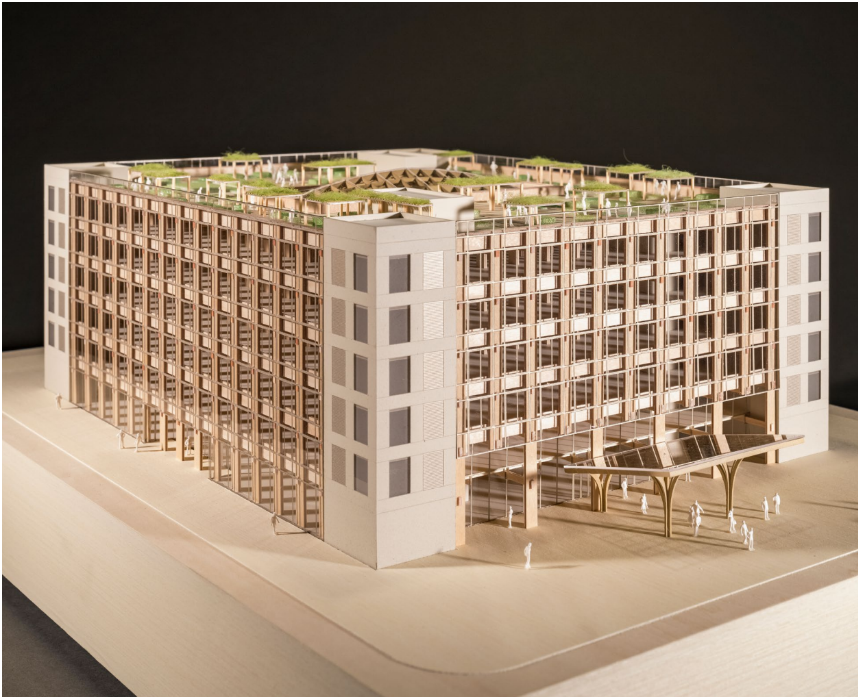
Design for reconstruction of Lviv hospital with the use of cross laminated timber as the primary material. Source: © Hiroyuki Hirai. https://shigerubanarchitects.com
